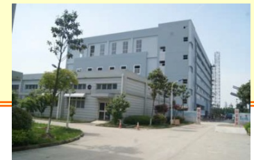
[Exterior of the plant]
