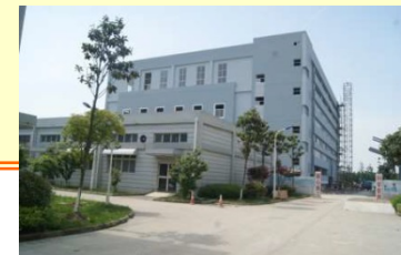
[Exterior of the plant]
