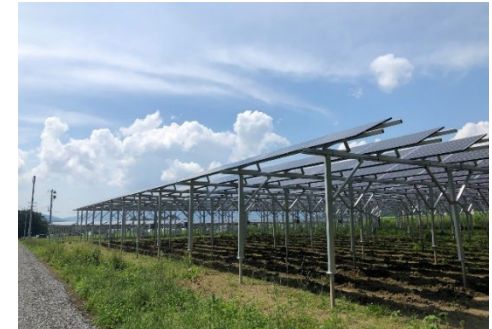
SBI Tono first solar sharing power generating plant (Tono City, Iwate Pref.)
