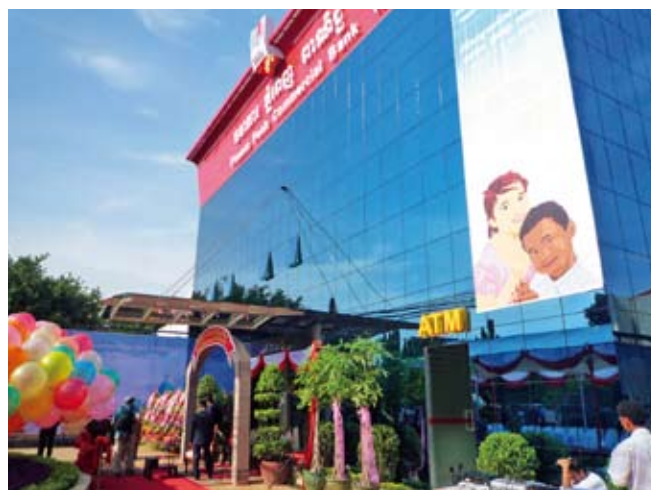
柬埔寨Phnom Penh Commercial Bank外观
